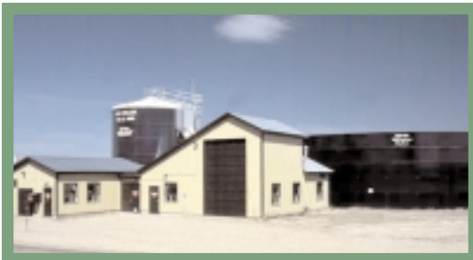
Complete Anaerobic Digester System
