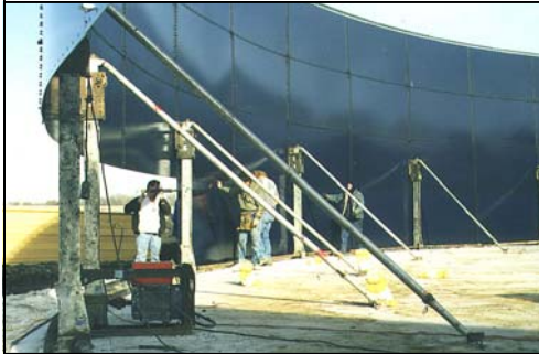
Typical E.S.P.C. jack-lifting tank during construction.
